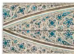
Vault of the Milan Cathedral
